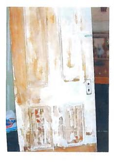
One time consuming (and back breaking), effort included the stripping and refinishing of all of the wood work in the house. Shown here a before (left) and after (right) picture is one of the solid chestnut doors that was taken to raw wood and refinished. Again this work is being done by volunteers.
